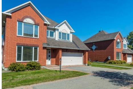
Figure 1: Canadian Centre for Housing Technology Field Monitoring Site in Ottawa, Ontario
