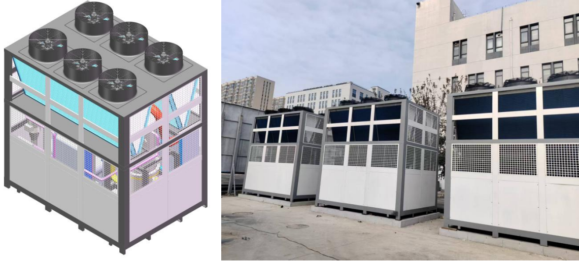
Figure 2. The MW level gas absorption heat pump unit.
