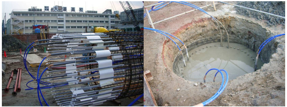
Photo 1. Energy pile system with cast-in-place concrete piles. Left: Four U-tubes tied onto the reinforced frame Right: Installation of four U-tubes in a concrete pile
