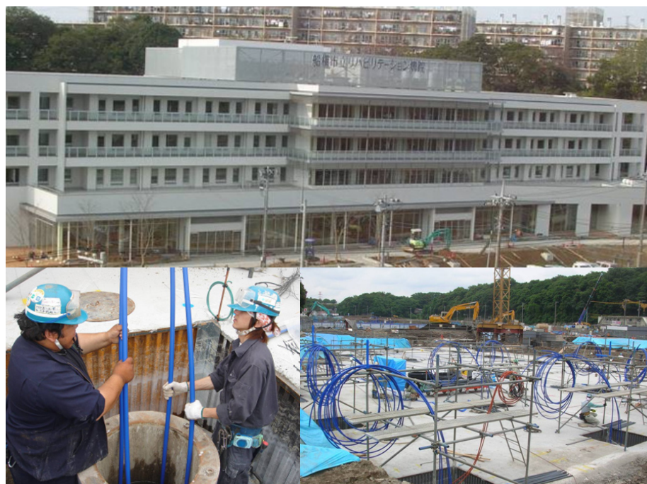
Photo 3. A closed system using pre-cast concrete piles in the Funabashi city rehabilitation hospital. Top: Exterior of hospital building. Left: Inserting two U-tubes in the hollow of a pre-cast concrete pile. Right: U-tubes from pre-cast concrete piles under construction.
