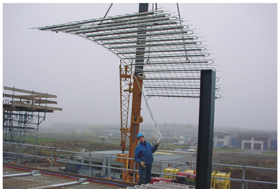
Figure 3 Prefabricated reinforcement mats for low-temperature floor loops.
