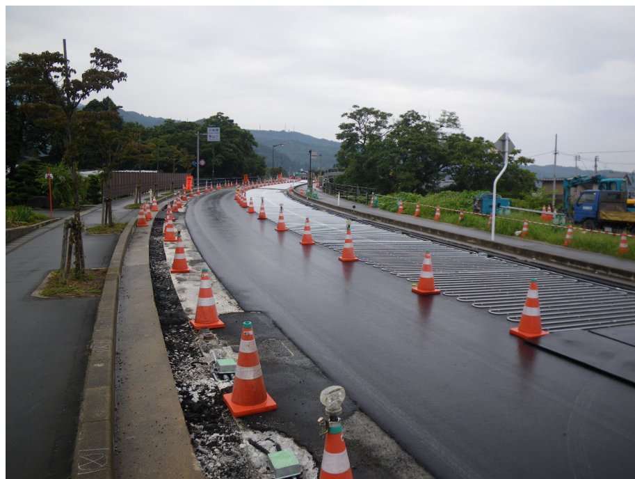
Construction site of Snow Melting System.
