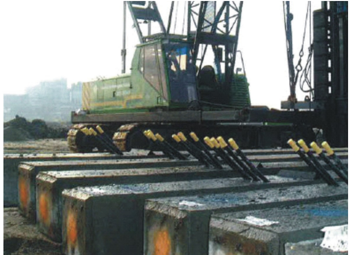
Figure 2 Piles with heat exchangers (left: Betonson, right: Voorbij). So-called 'energy-piles' are slowly gaining popularity in the Netherlands [6].
