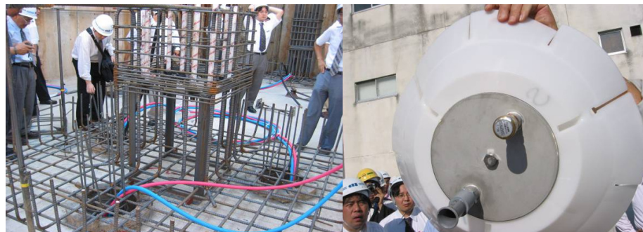
Photo 2. Tubing of the open system using the pre-cast concrete pile and a pile cap of the system in Fukui prefecture education center building. Left: Two tubes come from a reinforced frame of the footing. Right: A used pile cap.
