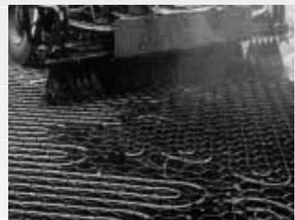
▲ Figure 2: Installation of the asphalt collector.
