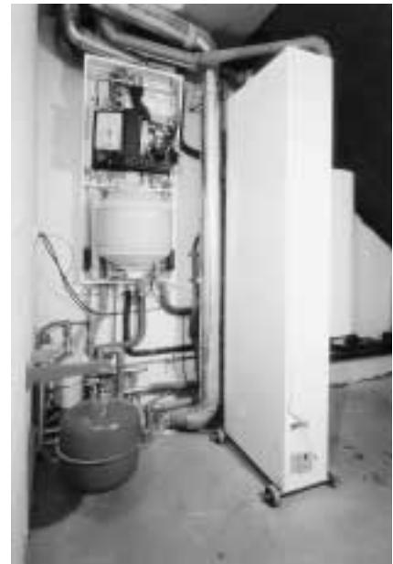
▲ Photo 1: The gas-fired heat pump (right) was supplemented by the HE central heating boiler (left) in the pilot project.
