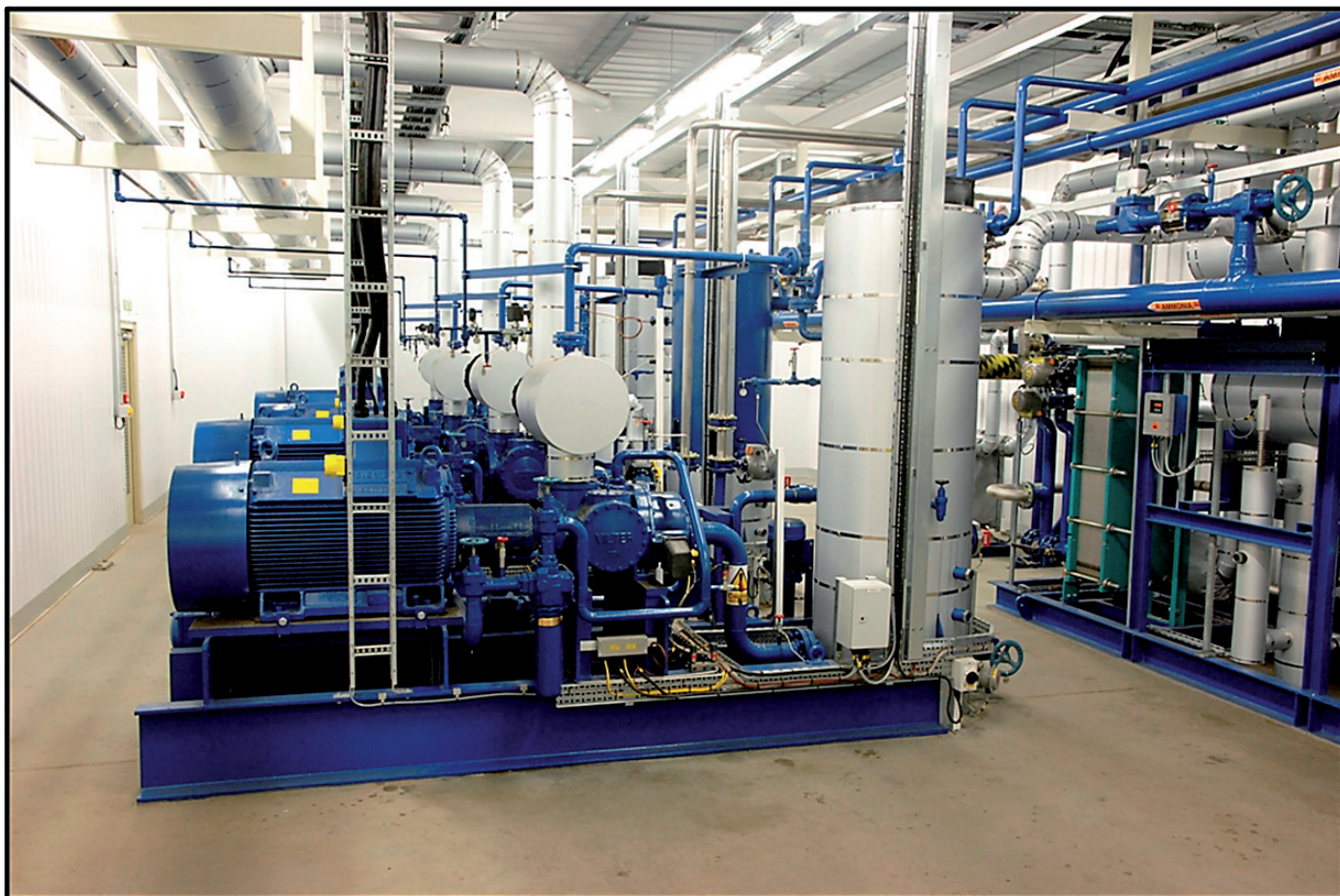
Figure 5 Self-contained ammonia heat pump for food processing
