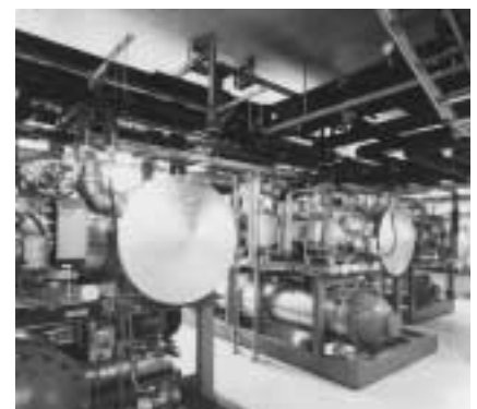
► Figure 2: Ammonia heat pump in a commercial building in Norway.
