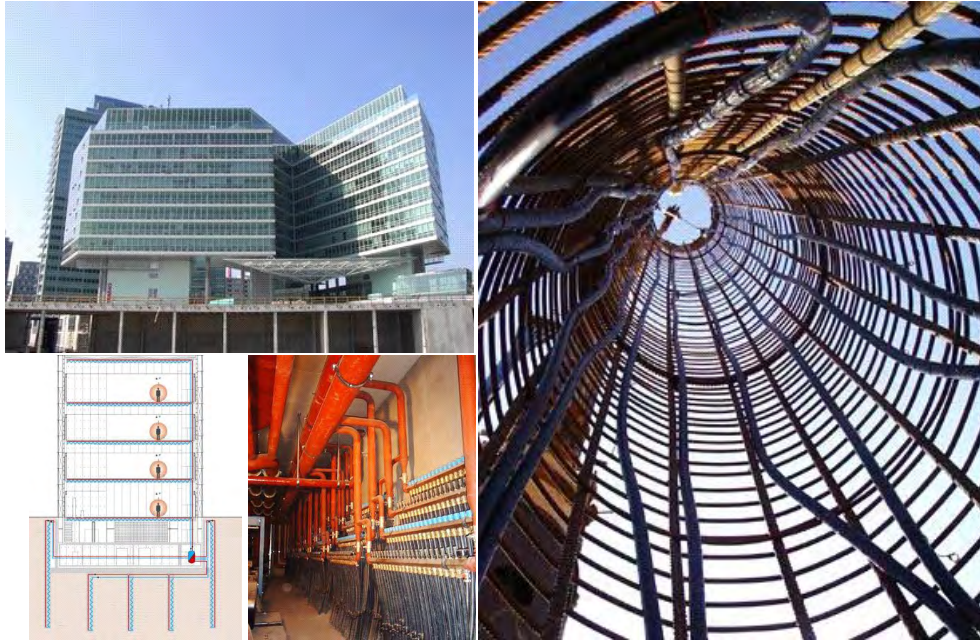
Fig. 5.29: Foundation piles as underground energy storage
