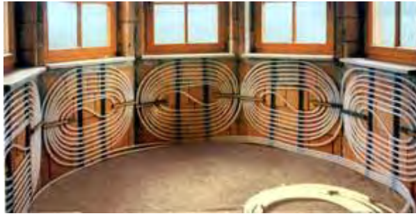
Fig. 5.13: Wall Heating System Supporting the Floor Heating System
