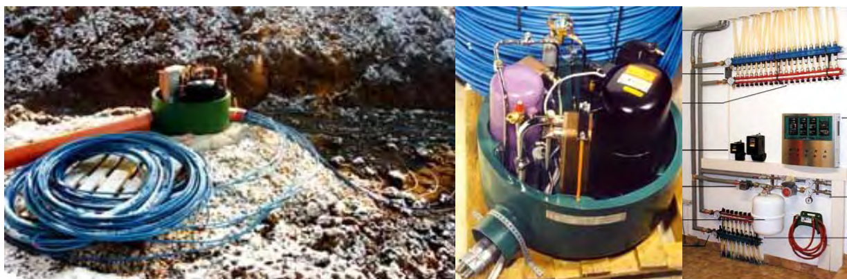
Fig. 5.22: Packaged DX Heat Pump with Propane as Refrigerant
