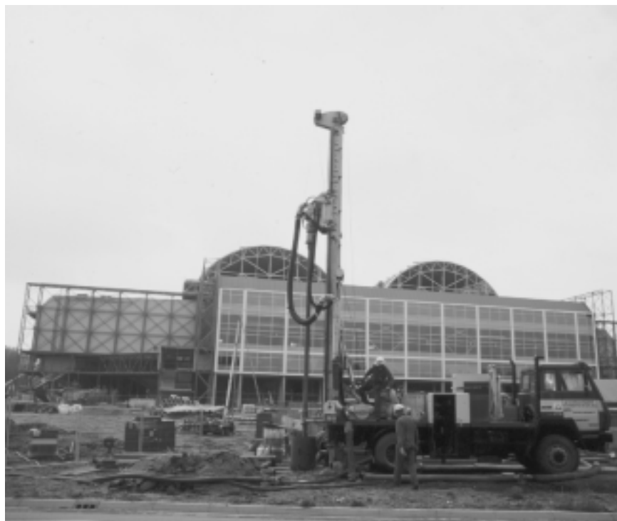
▼ Figure 2: Photo of the Gelredome stadium - installation of ATES.
