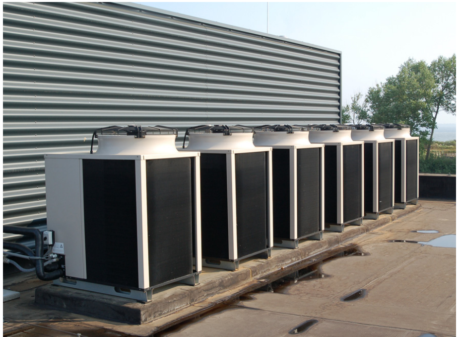
Figure 5. Cascade of six gas-fired absorption heat pumps heating a residential-care centre.
