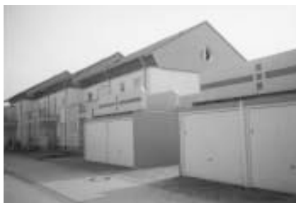
▲ Photo: Garages with concrete heat absorbers on the roof in a project in Waghäusel.
