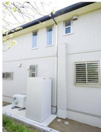
Annex 41: Field test installation of HPWH system combined with Solar thermal and PV collectors – Source: YAZAKI RESOURCES CO., LTD. Contribution to Japan Annex 41 draft interim report.
