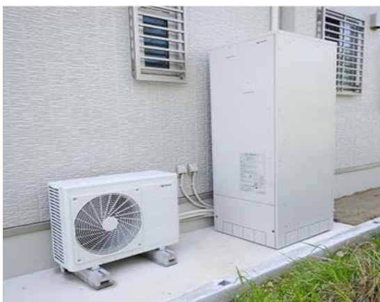
Annex 41: Field test installation of HPWH system combined with Solar thermal and PV collectors – Source: YAZAKI RESOURCES CO., LTD. Contribution to Japan Annex 41 draft interim report.
