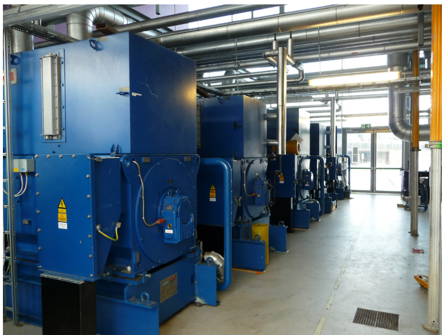
Drammen - high-temperature ammonia mono-screw compressor units (district heating)
