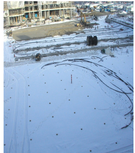
Figure 3. Borehole TES system at UOIT. Left: Present appearance, showing boreholes below university buildings. Right: View during construction, showing grid of borehole headers and interconnecting piping.
