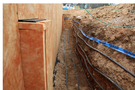
Figure 1. High density polyethylene tubing is placed against the outer walls of the excavation.
