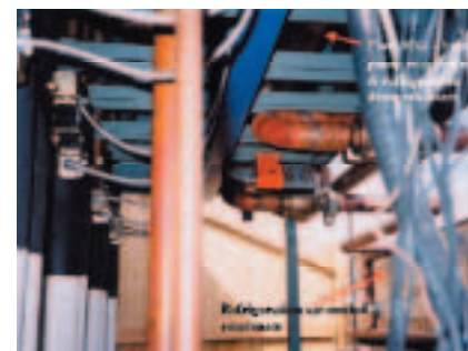
Figure 4: Plate heat exchangers (HX) for heat pump evaporators and refrigeration de-superheaters and sub-cooler at Canadian test store.
