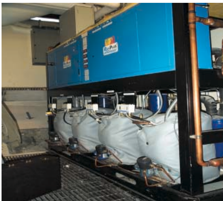
Figure 2: View of the compressor module of heat recovery heat pump
