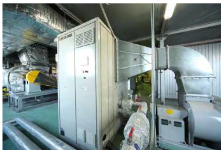
Figure 8-14: CO 2 heat pump air heater installation
