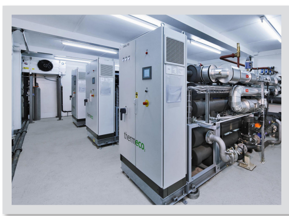
New CO 2 heat pump system for hot water generation and heating slaughterhouse in Zurich, Switzerland
