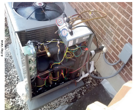
Annex 41: 2015 CCHP field test; single-stage vapor compression cycle with dual single-speed compressors – schematic (left image) and field test prototype system installed in late January at residence in Ohio. [Source: Oak Ridge National Laboratory and Copeland Compressor]
