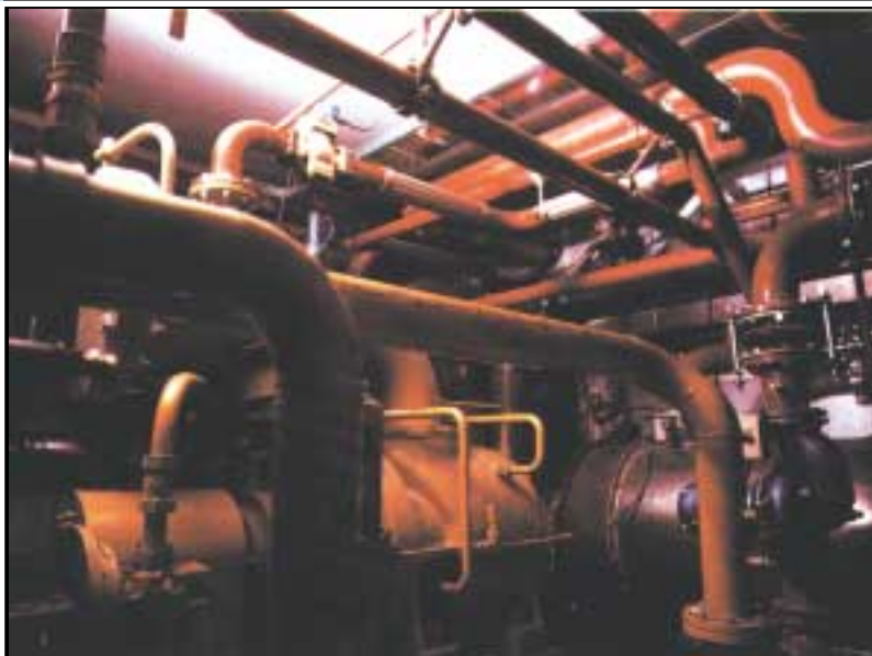
Above: Gas engine driven heat pump for the Amsterdam World Trade Centre.
