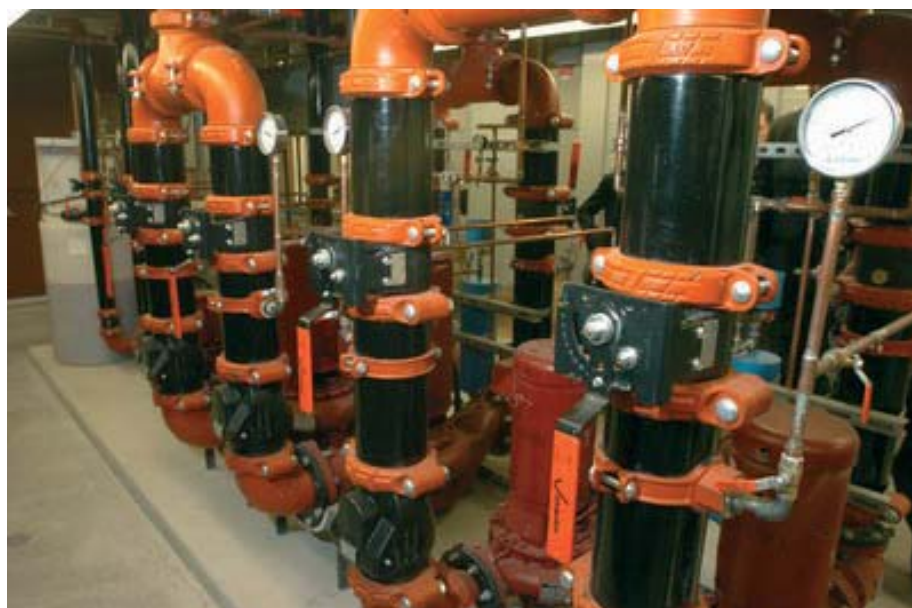
Figure 3: Secondary fluid pumping system for heat recovery
