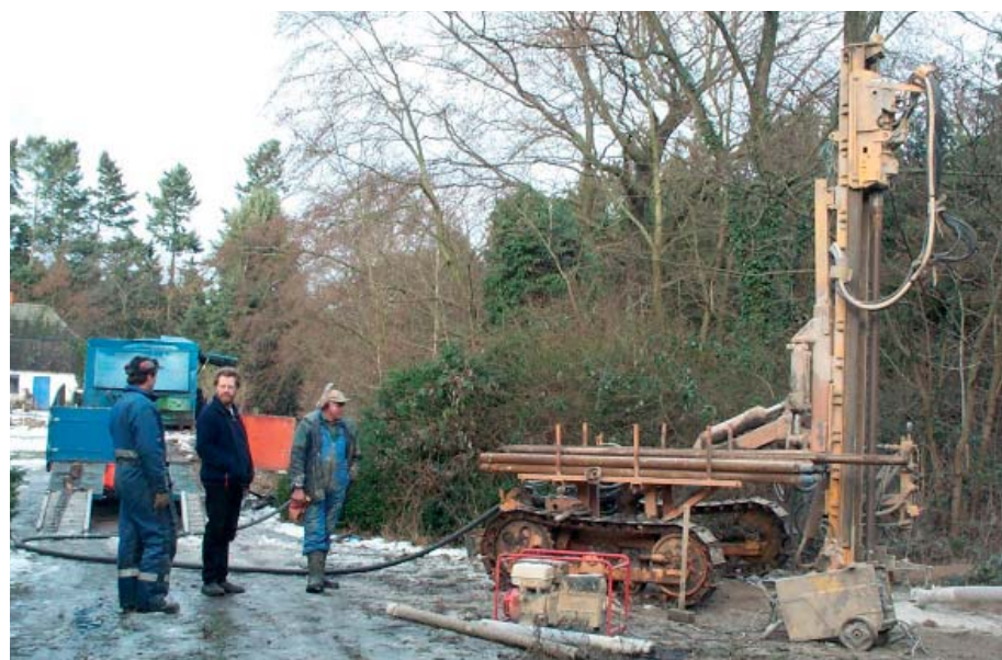
Figure 2. Drilling a borehole for a single family dwelling
