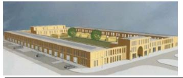
Project: Carré, Delfgauw, terraced houses. This concept realizes an energy performance coefficient of 0.6 with insulation levels (Rc) of 3.5 to 4 [m2.K/W], an Uc-value for windows of 1.2 [W/m2.K], balanced ventilation and ventilation heat recovery of 90%. The solar collectors add to the production of hot water and regenerate the ground source.
