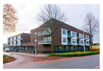
Project: De Tas. Biddinghuizen, apartments. An energy performance coefficient of 0.5 is realized with insulation levels of 3 [m2.K/W] for walls, floor and roof and Uc 1.2 [W/m2.K] for the windows. the calculation of the In energy performance coefficient, a 'normal 'value for the infiltration is used of 0,625 [dm3/m2.s]. The concept can be extended to include active use of thermal solar energy and photovoltaics.
