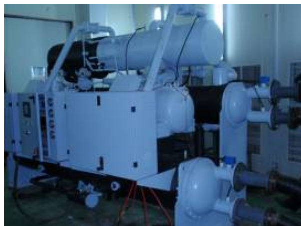
Figure 12: The Water-source Heat Pump Prototype
