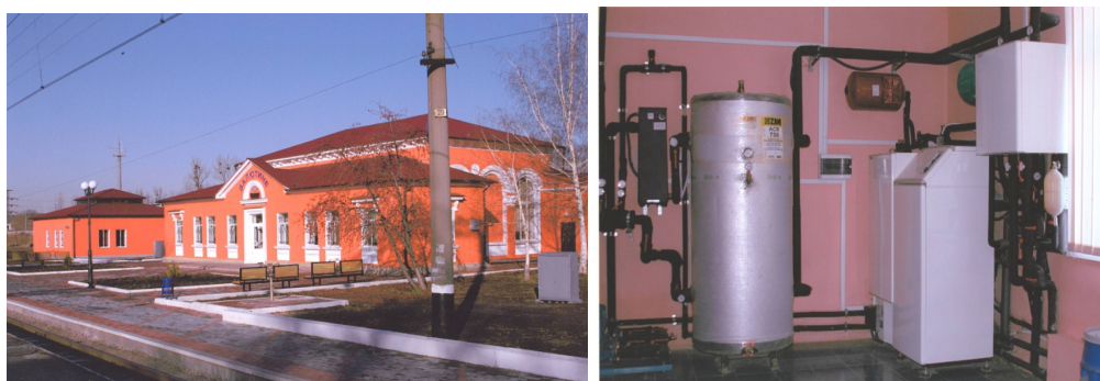
Fig. 6 Hot and cold water supply at Zalyutino station using geothermal heat pump a) station building, b) general form of heat pump boiler station.
