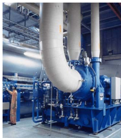
Figure 11: One of six 30 MW Sulzer heat pumps at the Stockholm district heating (1985) [www.friotherm.ch]
