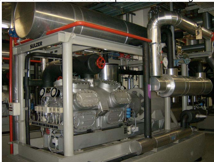
Figure 9: One of the four 440 kW heat pumps of the Lucerne railway station (1984) [Axima, CH-6010 Kriens]
