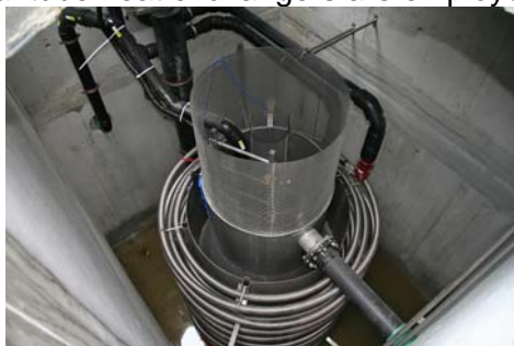
Figure 3: Wastewater collector with integrated heat exchanger. (Kalberer 2008).
