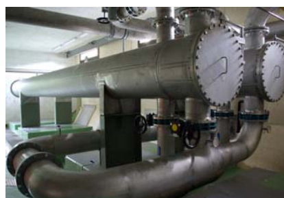
Figure 11: Heat exchanger in the WWTP of Berne: Power: 2x 700 kilowatt. (Wellstein J. 2007)
