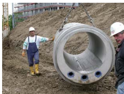
Figure 8: Sewer element with integrated heat exchanger (SwissEnergy 2005).
