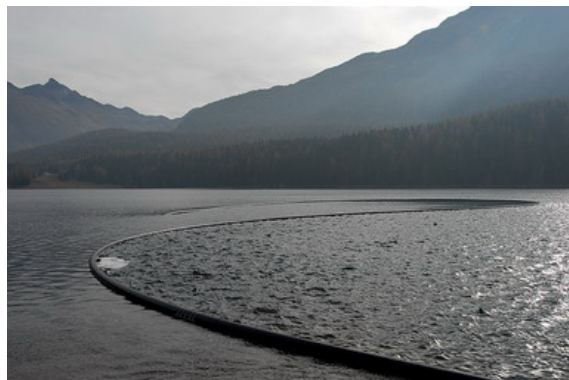
Figure 5: Lake water pipe prior to sinking
