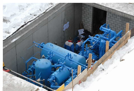
Figure 7: Building for heat pump
