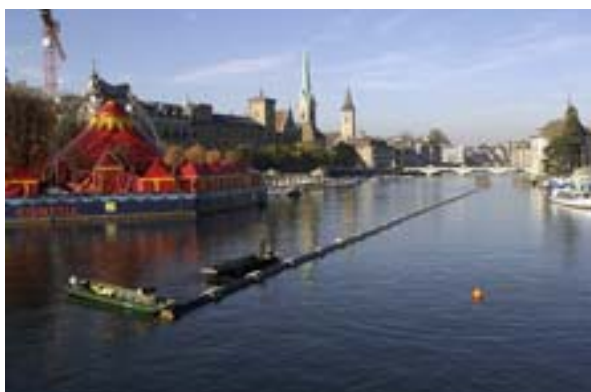
Figure 10: Lake water pipeline prior to sinking into the Limmat
