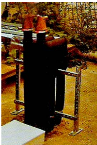
Figure 5: a) Brine cooler on the top of the earth probe
