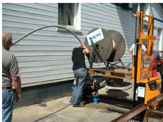
Figure 3: a) Inserting the 50 m heat pipe at Kaeltro
