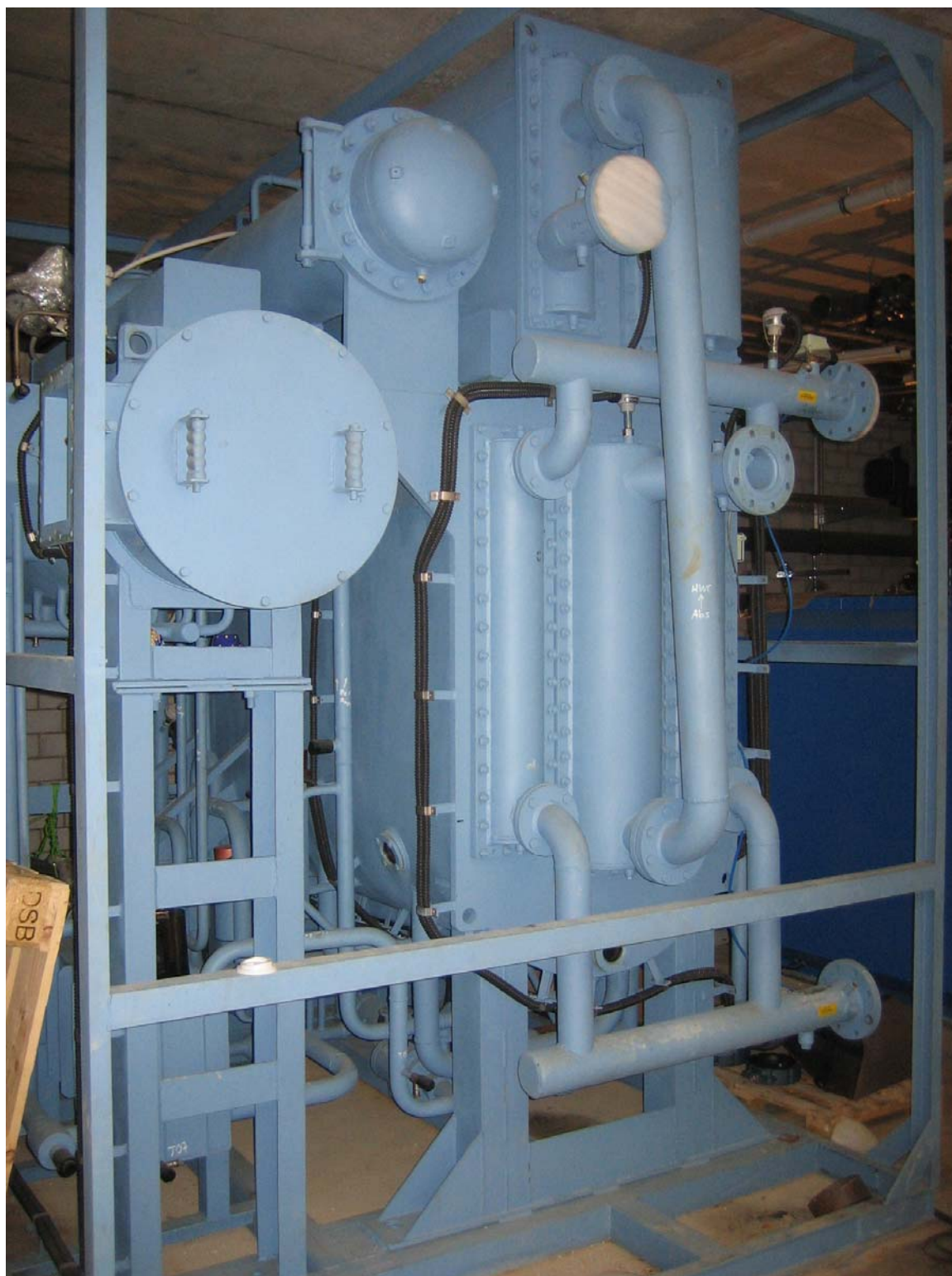
PHOTO 1: Exhaust fired Single-Double effect Absorption Heat Pump at KONSTANZ, GERMANY
