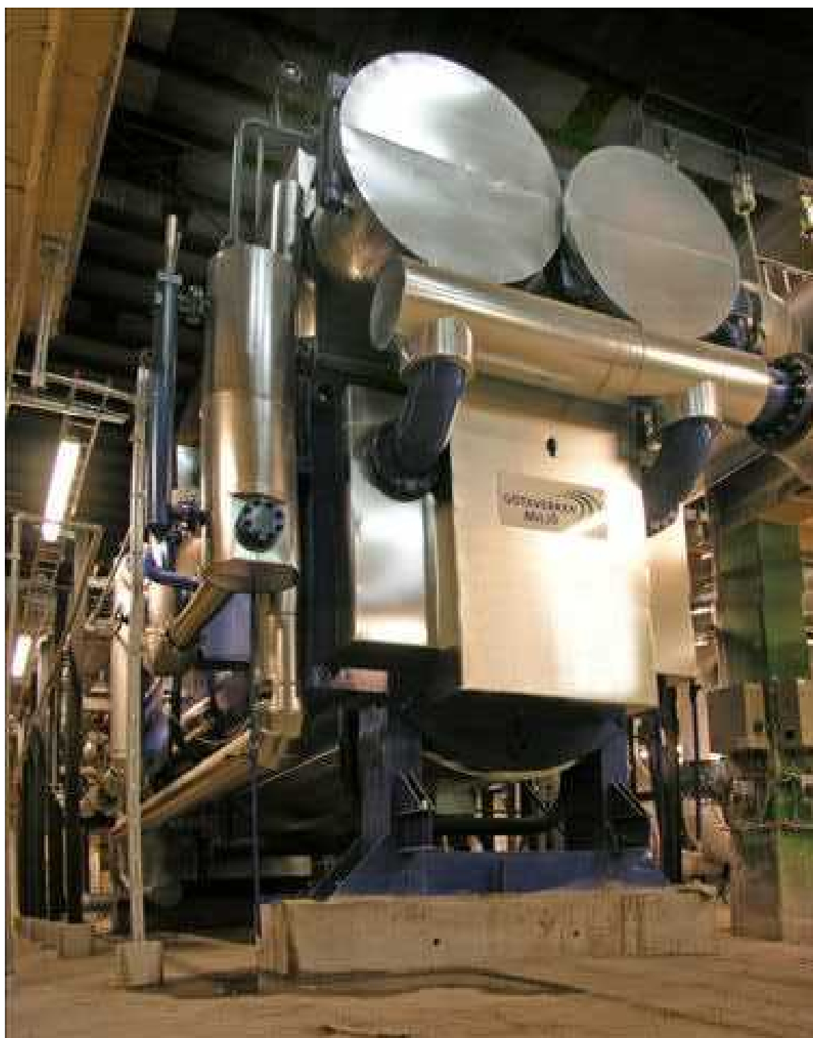
PHOTO 3: Steam driven 13 MW AHP at Vestforbraending Copenhagen, Denmark
