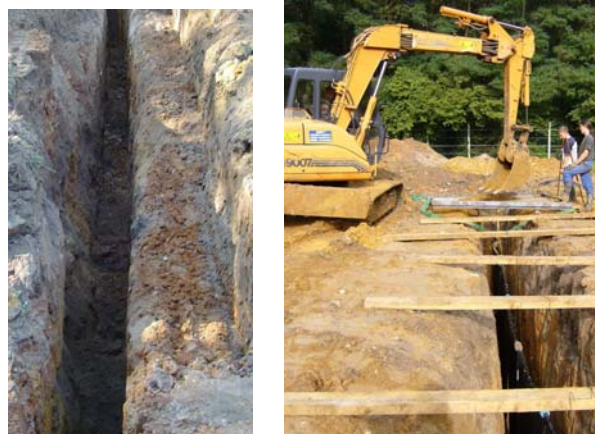
Figure 6 : Trenches drilling and filling up
