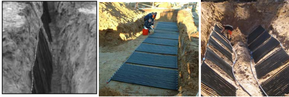
Figure 2 : Vertical, horizontal and V-trenches installations
