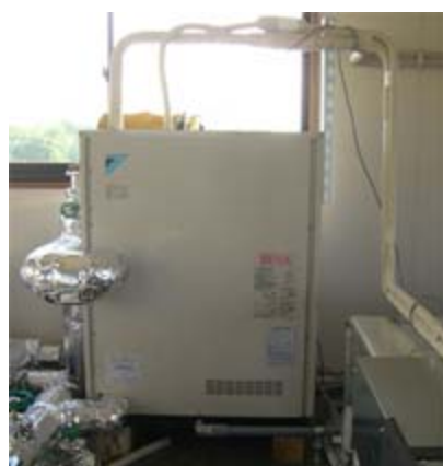
Figure 6: Appearance and specification of water source multi-split heat pump unit
