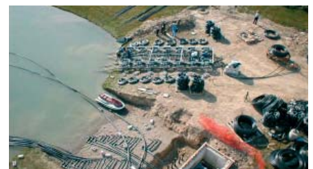
Photo: courtesy of Lane Brown, Geothermal Designs Associates, Inc. Fort Wayne, Indiana – Plastic pipe coils fabricated as a pond loop
