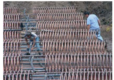
Copper pond loop constructed and installed on the golf course in Oklahoma - 2005
