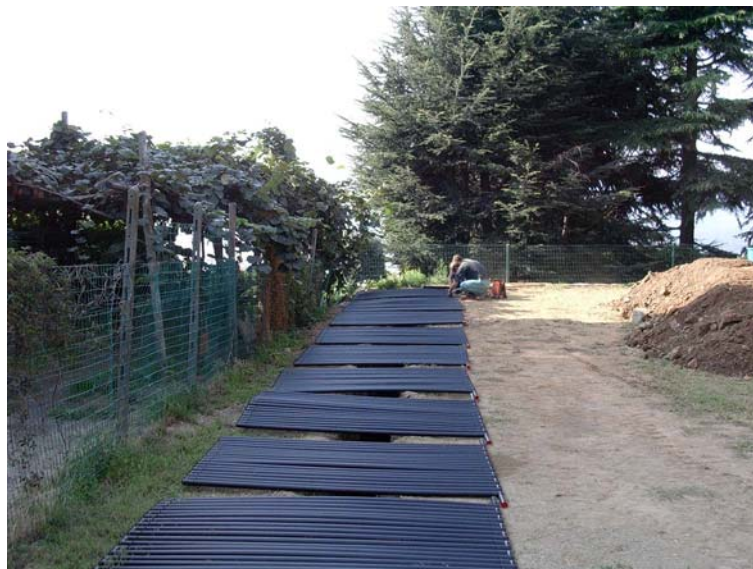
Figure 2: “Compact collectors” installation
