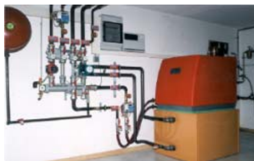
Figure 3: Heat pump Dimplex/Siemens (Type WI 15C)
