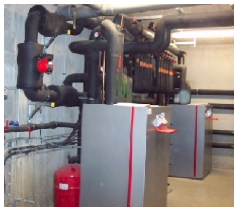
Figure 6: Brine-to-water heat pumps
