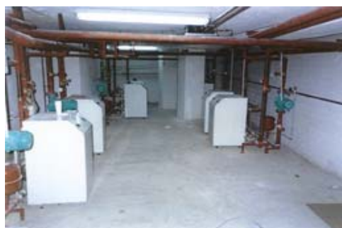
Figure 8: Heat pumps installed in the basement
