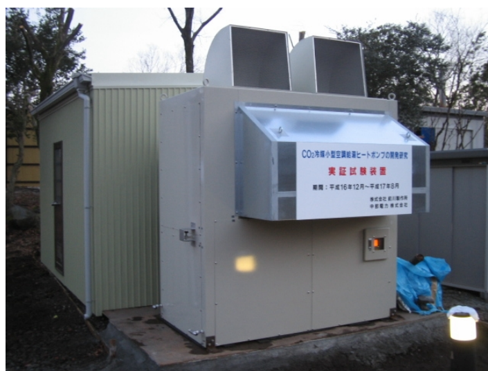
Figure 6: the Developed Heat Pump Installed at a Tourist Hotel
