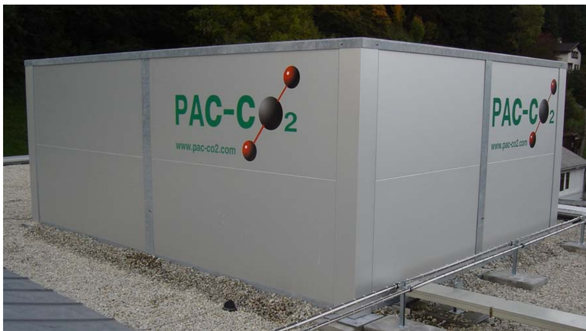
Figure 3: CO 2 heat pump to produce hot sanitary water for a hospital [Anstett 2006]
