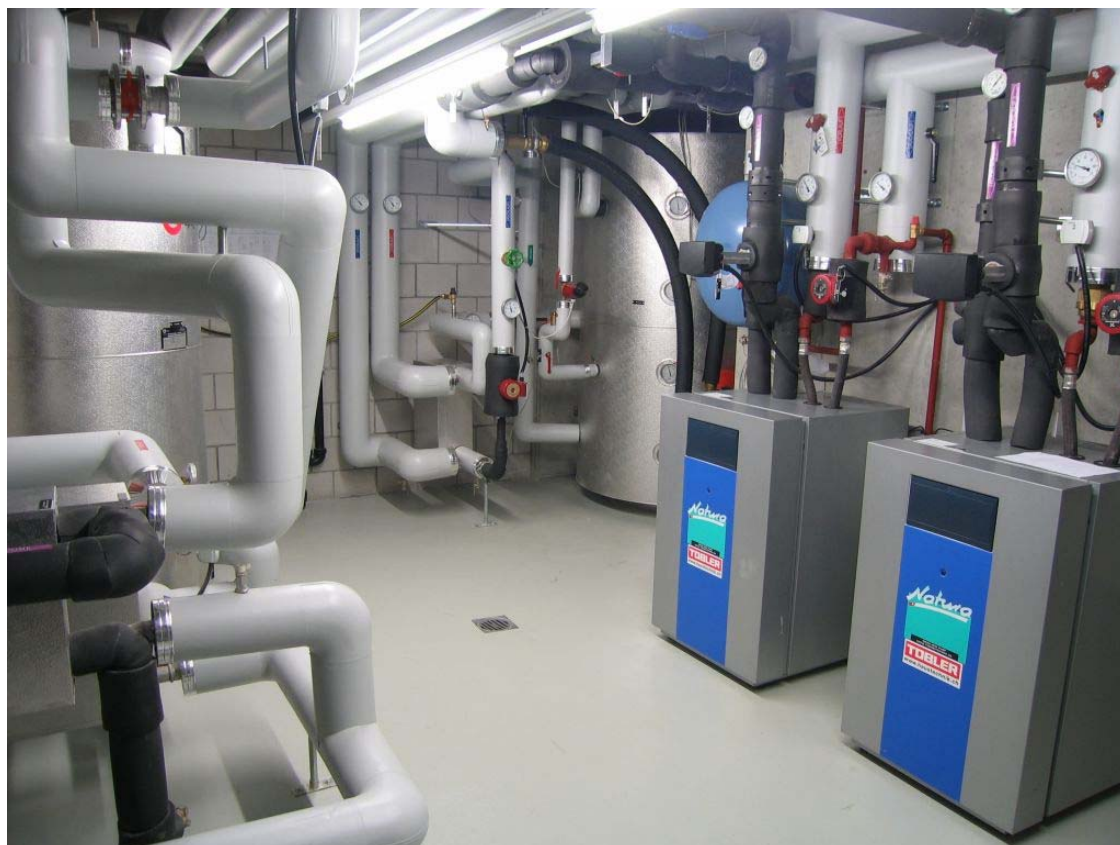
Figure 5: Heating room [Gabathuler et al. 2007]. At left storage tank, at right heat pumps
