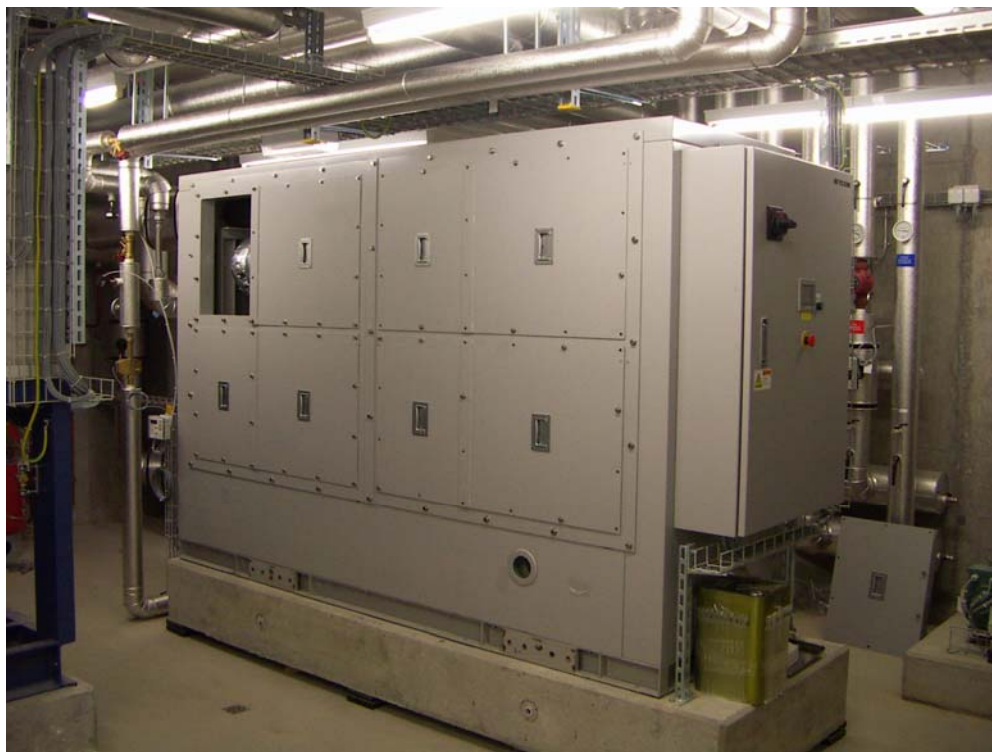
Figure 8: Heat pump package installed in Switzerland
