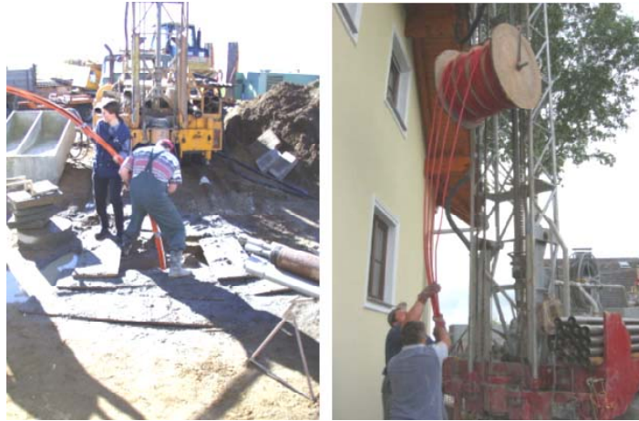
Fig. 8. Installation of the probes (left: one of the first installations; right: standardized)
